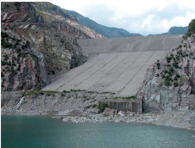
Above, top: Figure 4 – Damaged concrete slab of concrete face rockfill dam detected after the first filling of the reservoir; Figure 5 – Erosion damage at dam toe (left) and concrete protection in plunge pool after operation of the tunnel spillways (right)
